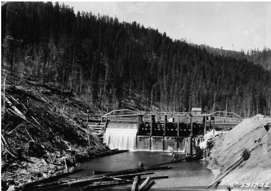
Figure 14.4. A splash dam on the North Fork Willamette River, 1924. Loggers stored water behind dams like this one and released it to carry logs downstream. U.S. Forest Service photograph by T. H. Gill. Public domain.
