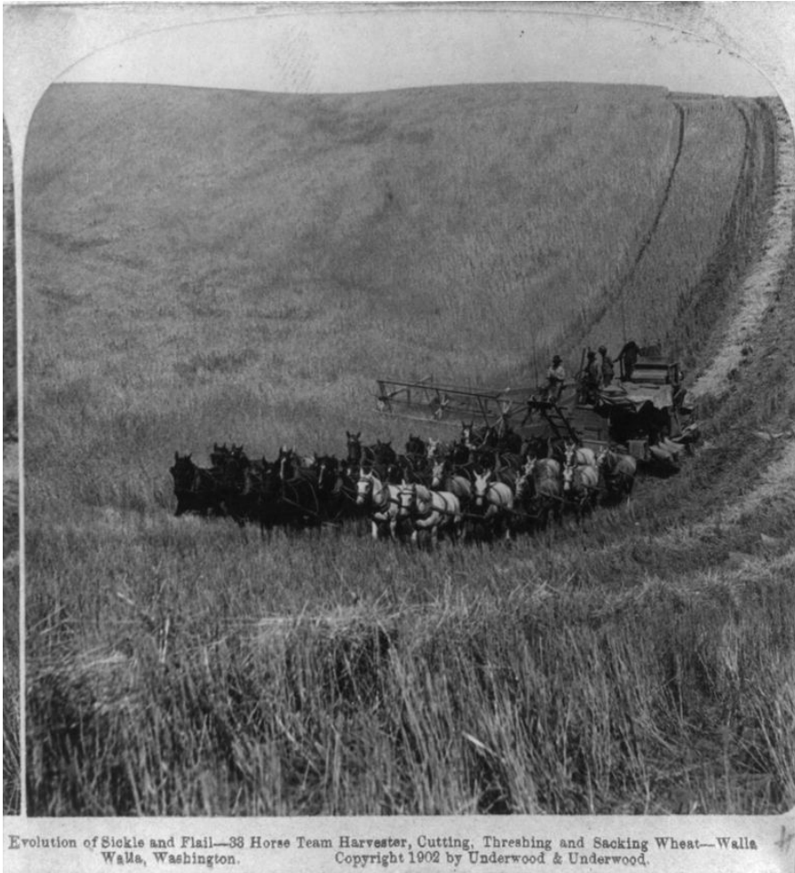
Figure 15.5. A combine drawn by 33 horses, cutting, threshing and sacking wheat near Walla Walla, Washington, 1902. One machine did three jobs, pulled by a field full of horses. Underwood and Underwood stereograph, Library of Congress. Public domain.
